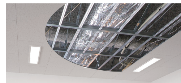
Our own anti-seismic ceiling construction technique
