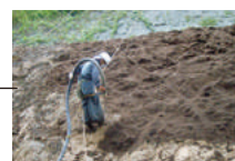
Greening by spraying work
