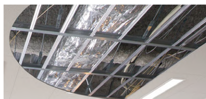
Our own anti-seismic ceiling construction technique
